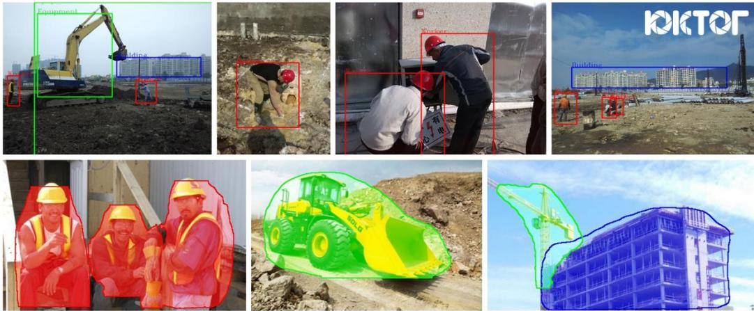
**Figure 3. Detection of building (blue), equipment (green), and worker (red) by YOLO (top row) and Mask R-CNN (bottom row) algorithms.**
