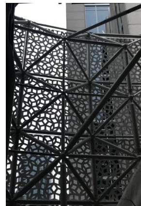
Interior view with traditional spaceframe
